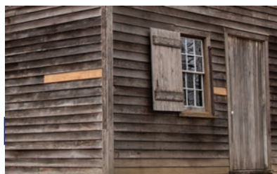
Siding removed to test stains and finishes.
