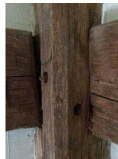
Pegged, timber frame construction
