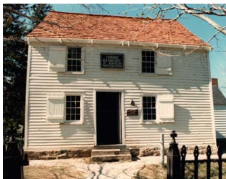
Meeting House ca. 1978, with new shake roof and before the paint was stripped
