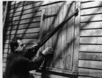
Hanging the restored shutter.
