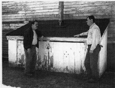
Paul Basile & Jim Brotherton discuss the removal of the shed on north side when new heating system is installed.
