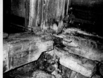
Additional work is needed on the vertical support post and sill..
