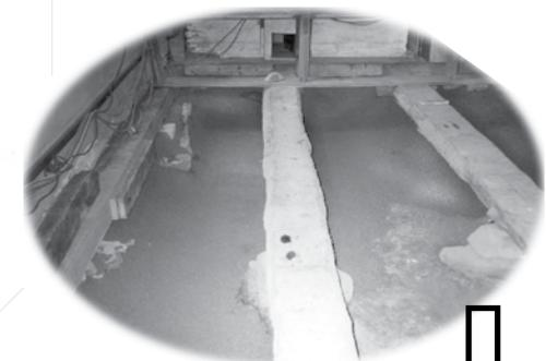
Remove floor; clear debris; level ground; repair and reinforce floor beams; pour cement vapor barrier.
