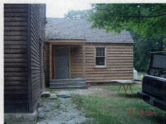
Annex, waiting to be stained
