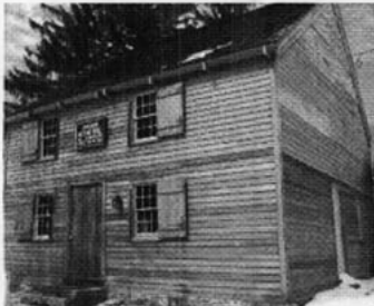
Front & East side , sanded & treated with linseed oil.
