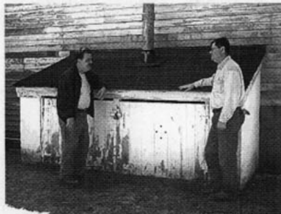
Paul Basile & Jim Brotherton discuss the removal of the shed on north side when new heating system is installed.
