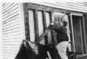
May '03 - South Wall Restoration
