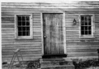
Nov., 2003 - South Wall Door Trim & siding restoration completed
