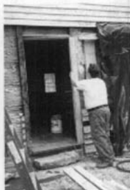
May '03 - East Wall Side Door Trim Restoration
