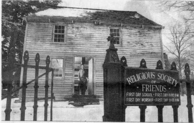
Hal Haydock stands in the doorway of the meeting house. Exterior paint stripping completed and ready for linseed oil finish in spring of 2004.
